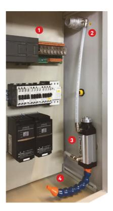
The VRX-500 cooler (fig.1) is actuated with compressed air from outside; the flow of cold air is directed, by using adjustable nozzles, on the electrical components that give off the most heat, while the exhaust of hot air is channelled by the red hose (fig. 3) to actuate the AM Series amplifier
